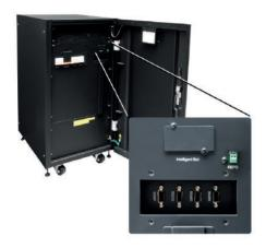
The Triton has extensive front accessible communication interfaces (eg 10-20 kVA).
