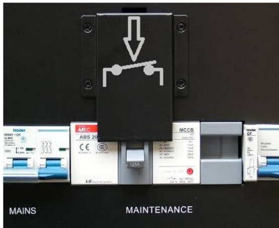
Fig. 6-1 Correctly placed safety cover for the manual by-pass (example illustration).
